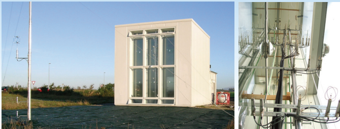
Hot-sphere anemometers placed in the double-skin façade.
