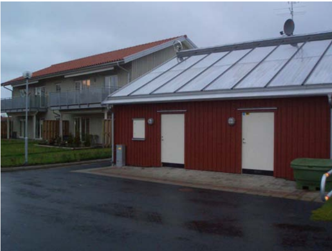
Figure 4. Passive houses at Frillesås with technical house containing solar heating system. Photo: Inger Andresen.
