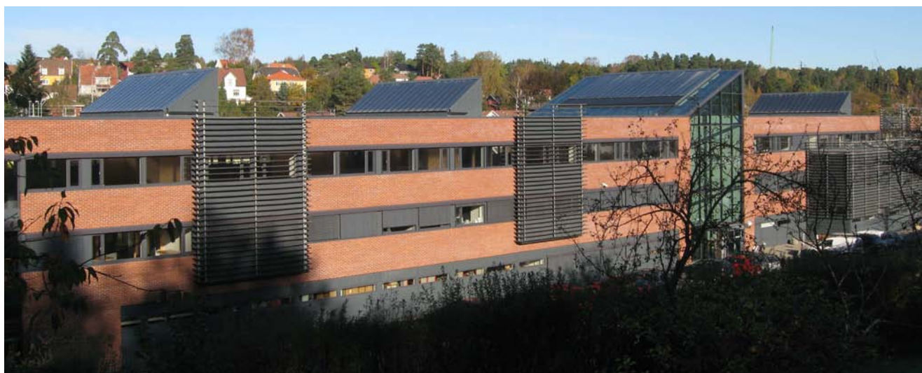
image 1 Bravida building east facade
