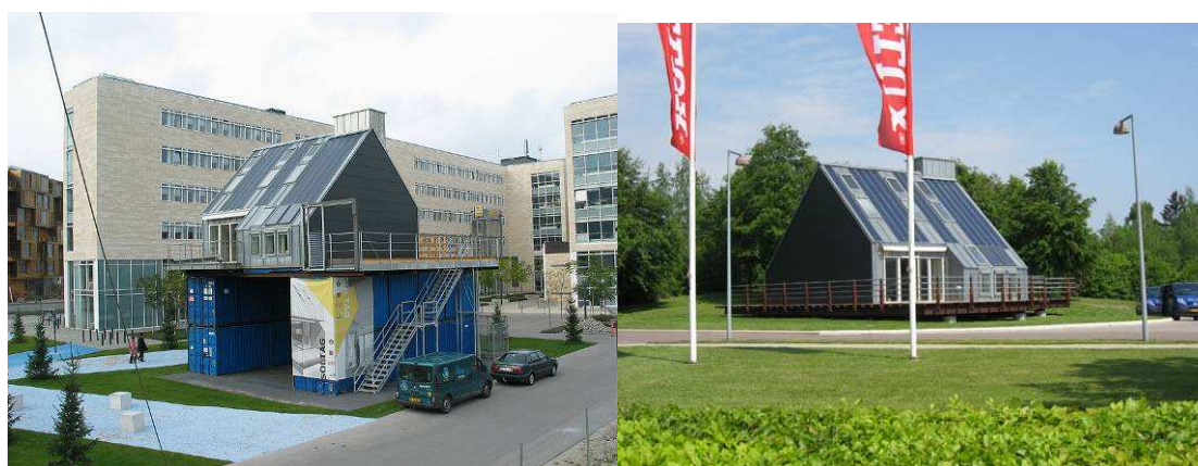
Fig. 2.1. Prefabricated SOLTAG CO 2 neutral rooftop dwelling exhibited in Ørestad, Copenhagen from August 2005 till the spring 2006. It is now situated at Velux headquarters in Hørsholm.
