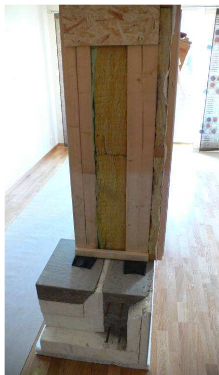
Figure 3 Wall and ground construction.
