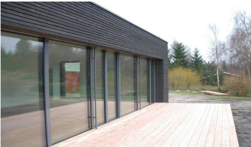
South-west elevation with terrace
