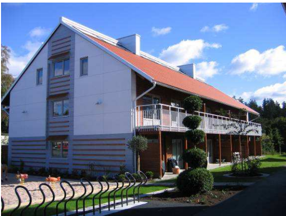
Figure 1: Apartment building in Värnamo, Oxtorget
