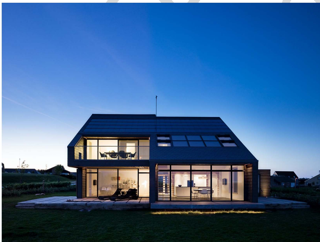
Fig. 1. Home for Life: the south-facing smart window facade, the roof with integrated roof top windows, solar cells, solar heat panels, and the weather station on top of the roof. Photo by Adam Mørk.
