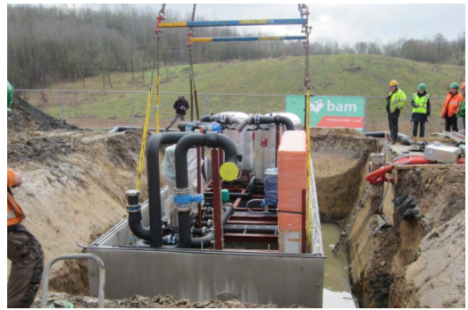
Figure 12 – Putting in place of the minewater installation production well
