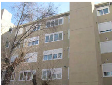
Figure 15 – Rehabilitated building – West façades
