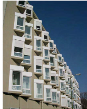
Figure 13 – Renovated building – East façade
