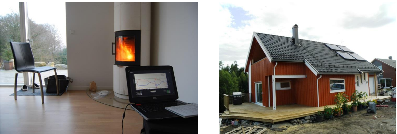
Figure 2. Auto-pilot wbs in a brand new house in Skaderborg/Denmark (left) and hydrostove with solar heating in Langhus/Norway (right).
