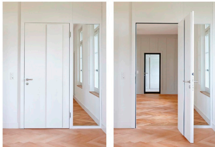
Figure 5. Active overflow system as a so-called “Verbundlüfter” by the company Erich Keller integrated into the door leaf in the listed manor house Brännengut in Bern (Switzerland).
