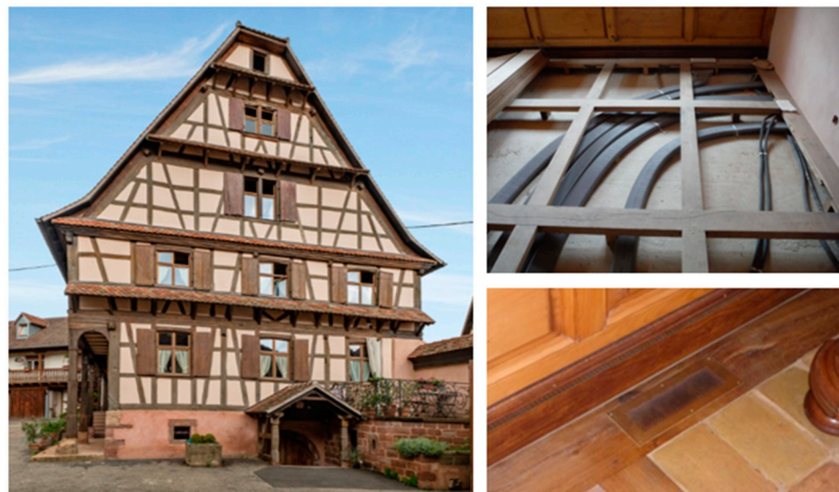
Figure 2. One of the documented examples. A timber-framed house from 1783 in Schnersheim, Alsace, France: Architecture, a “hidden” air supply, ventilation ducts of the HRV in the floor. Source: Denis Elbel.
