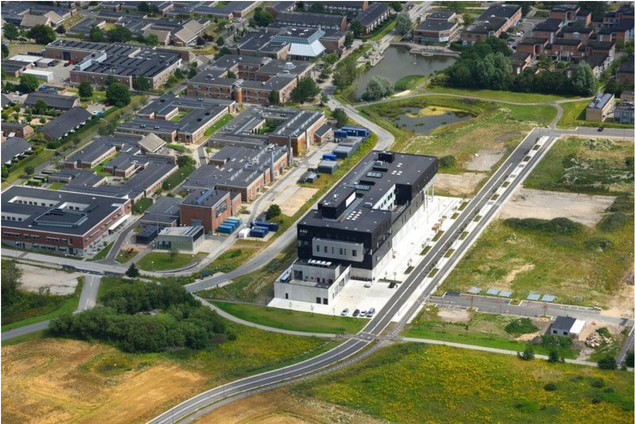
Figure 10: Aerial view of the TMV 23 building in its surrounding environment on the Aalborg University main campus. The South façade, the West façade and the roof of the building are visible. In 2022, a new building was built on the East side of the TMV 23 building (the upper right corner of the TMV 23 building in the picture) but was not visible yet in that aerial view (credit to Aalborg University).
