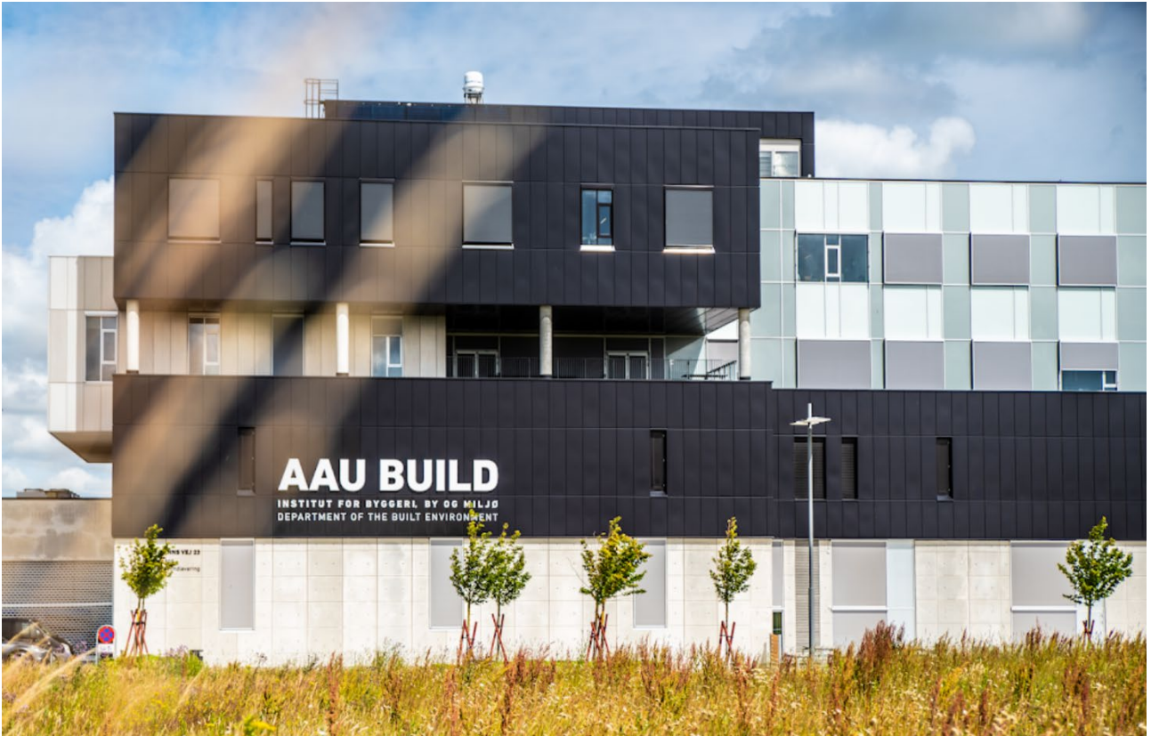
Figure 5: View of the South facade of the TMV 23 building (credit to Aalborg University).
