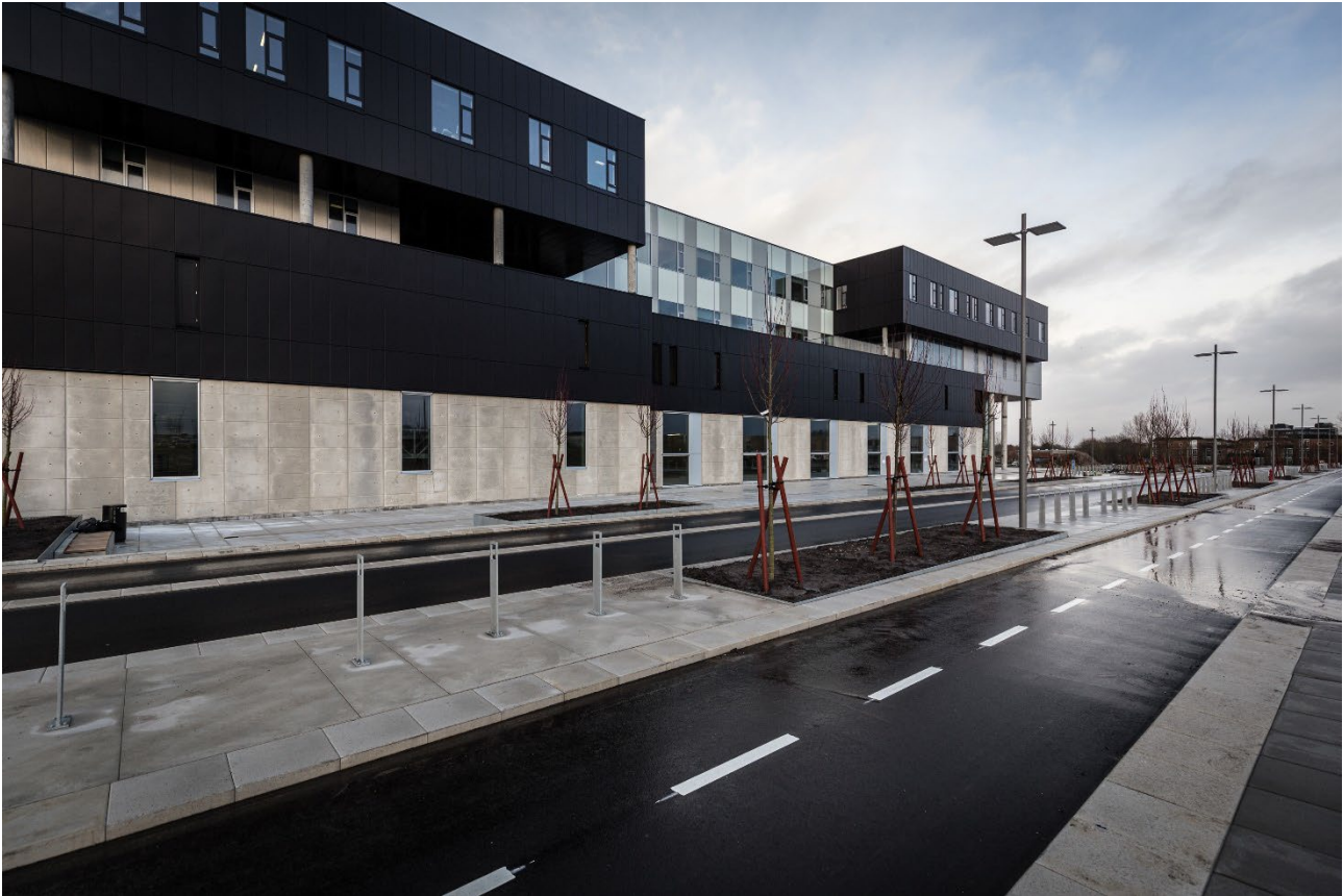
Figure 6: View of the South facade of the TMV 23 building (credit to Ronge Fotografi).
