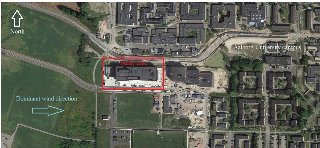
Figure 3: Aerial view of the TMV 23 building in its surrounding environment on the Aalborg University main campus.
