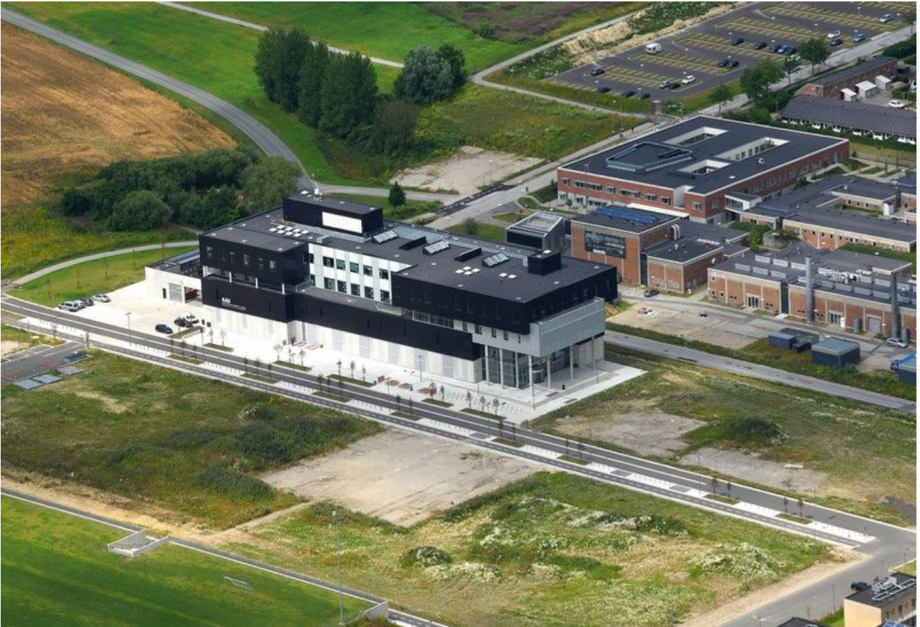
Figure 11: Aerial view of the TMV 23 building in its surrounding environment on the Aalborg University main campus. The South façade, the East façade and the roof of the building are visible. In 2022, a new building was built on the East side of the TMV 23 building (the right side of the TMV 23 building in the picture) but was not visible yet in that aerial view (credit to Aalborg University).
