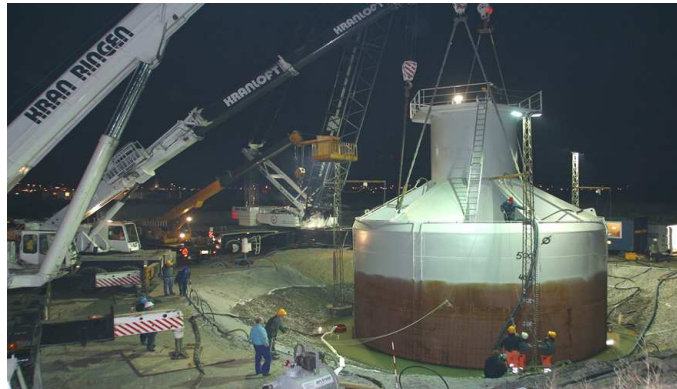
Figure 7: Real-scale installation of a monopod bucket foundation in Frederikshavn, Denmark
