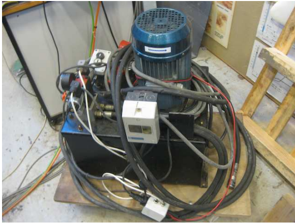
Figure 12: Hydraulic motor and cables
