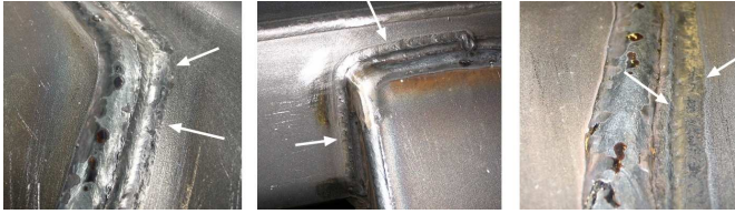
Figure A.18: Examples of final production quality TIG dressing, free from undercutting and significant imperfections.
