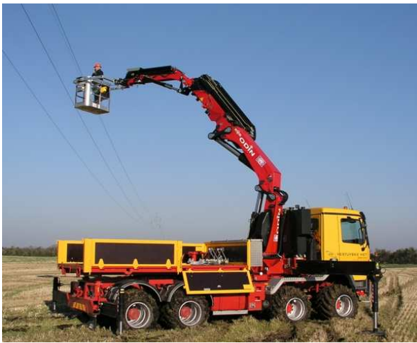
Figure E.1: Truck with loader crane used for personal lift.
