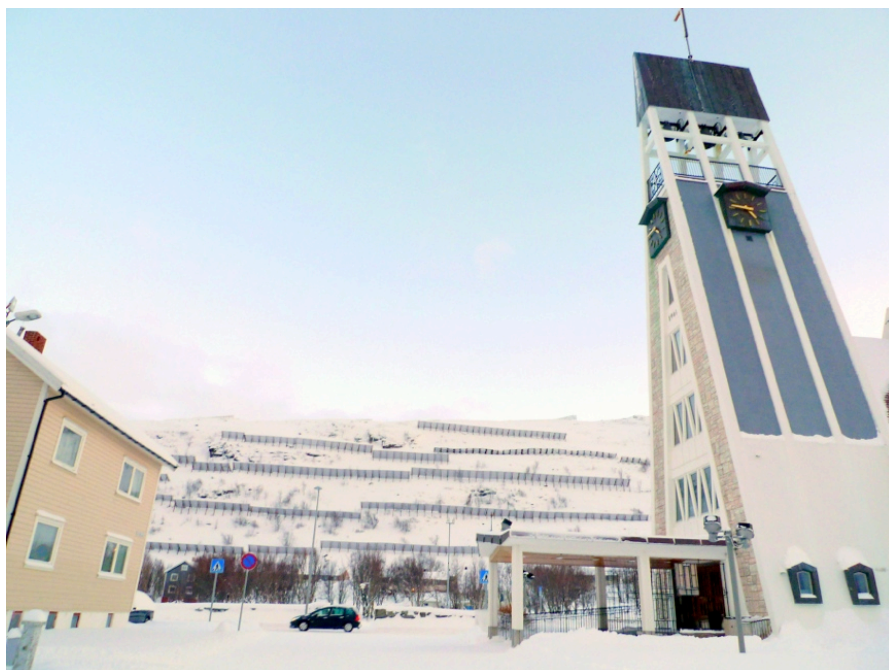
Even the church needs protection from avalanches in Hammerfest. Photo: H. Dannevig
