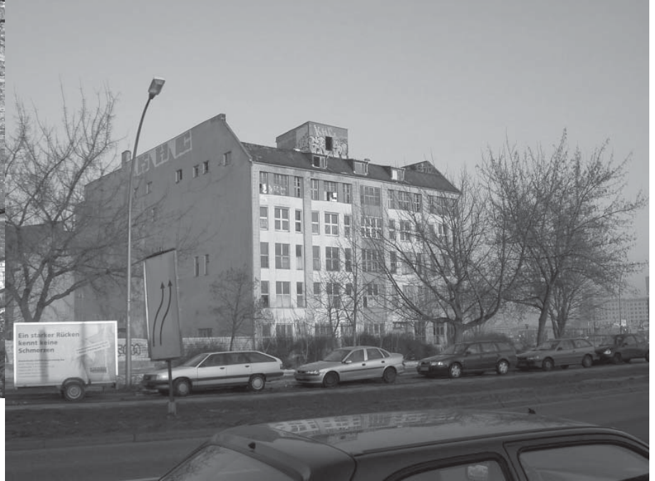
Fig. 5 and 6: The economical problems of Berlin is especially evident in the former East Germany (Photo: Lea Holst Laursen)
