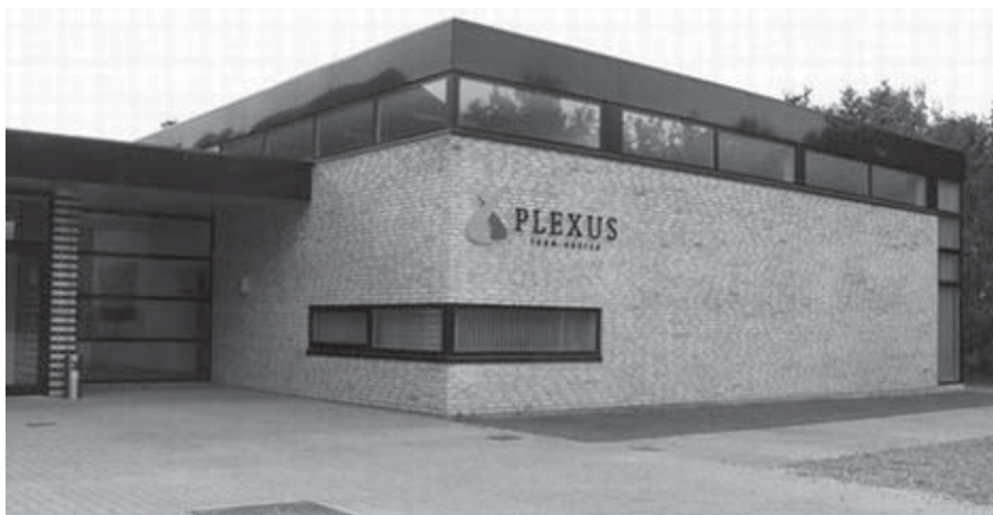
Fig. 122: The new community center in Idom-Raasted (Photo: Idom-Raasted, 2008)
