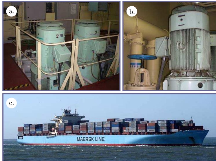
Fig. F.1: The cooling system SW pumps (a.) and LT FW pumps (b.) onboard the 6500 TEU container vessel "Maersk Senang" (c.), from which the experimental data is obtained.
