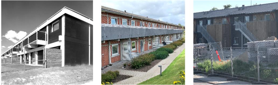
Figure 101. Images of two major renovations of case C: the hitherto appearance (middle) and its current ongoing transformation (right). (First image of original facade (left): courtesy by Aalborg Stadsarkiv. Photo 1966 by J. Brems)
