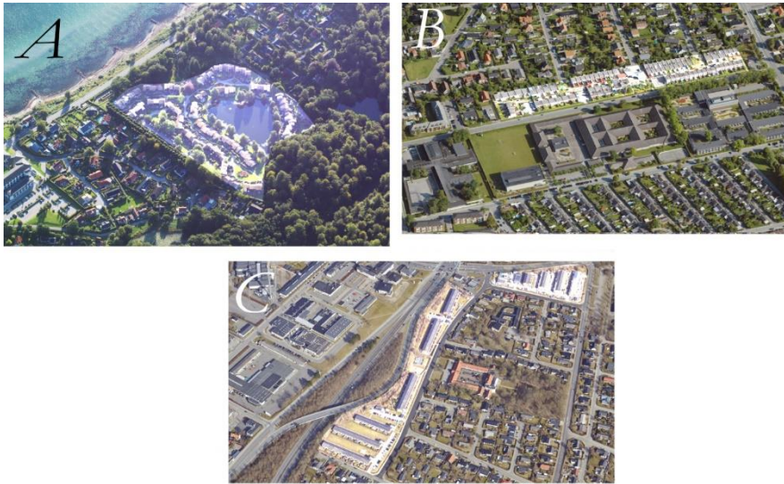
Figure 96. Case A. Sjølund (top left), Case B. FlexiBo (top right), Case C. ConBox (bottom) Courtesy of “Styrelsen for Dataforsyning og Effektivisering” (SDFE).
