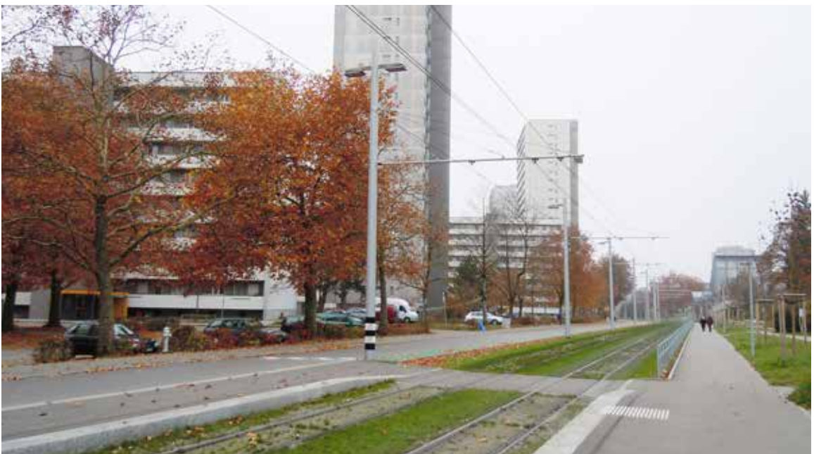
FIGURE 1+2: First impressions of Bern light rail. Above: the central node at the rail way station where the light rail network integrates with the regional network. The roof is shapes like a wave connecting the nodes. Below: The new light rail corridor in the midernistic housing area in Bern West (Photos by author).
