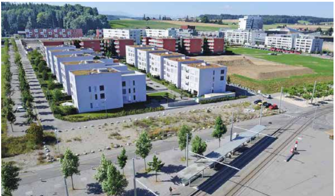
FIGURE 9+10: Above: The design of the light rail line has been created through a site specific approach where the unique character of each stops has been the basis for each design. Below: Ansermetplatz a new connection between the existing quarter Gabelbach and the new quarter Brünnen (Source: Dossier Stadtraum 2012).
