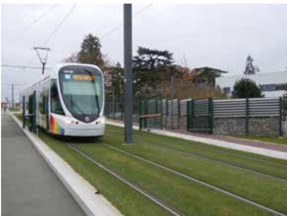
FIGURE 15: 70% of the route is green tracks. It was a political decision to construct the green tracks. This is to reflect the agricultural history of the area, and the identity as a green and agricultural area. (Photo by author).
