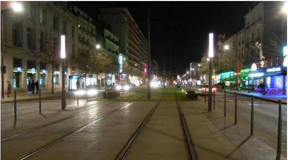
FIGURE 1+2: First impressions of the light rail corridor at Boulevard Foch in Angers city centre. Above: the rainbow image in motion. Below: The green tracks (Photos by author).
