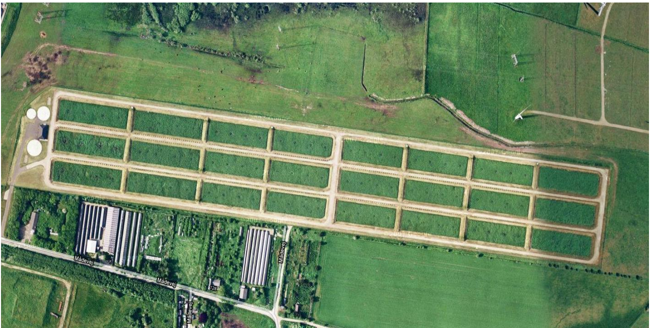
Figure 2. Reed bed facility located in Esbjerg, Denmark. It is composed of 24 basins, each of approx. 2200 m 2 . Storage tanks are visible left of the basins.
