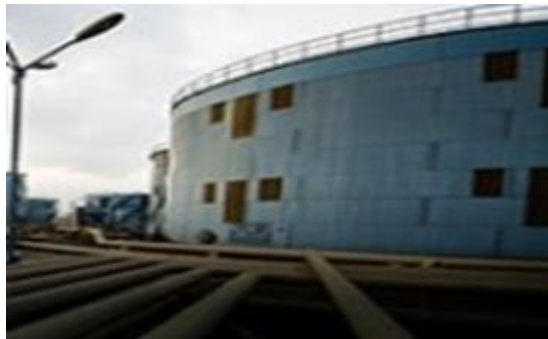
Figure 6-2 Storage capacity of PSOs products
