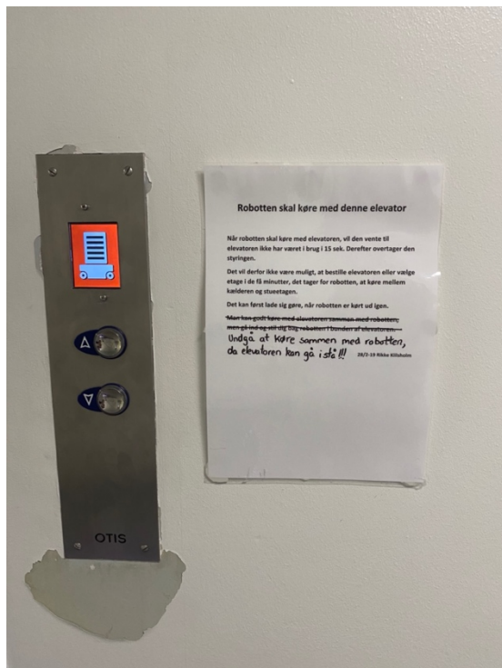
Figure 38 Robot in charge of elevator, at OUH, hence the symbol
