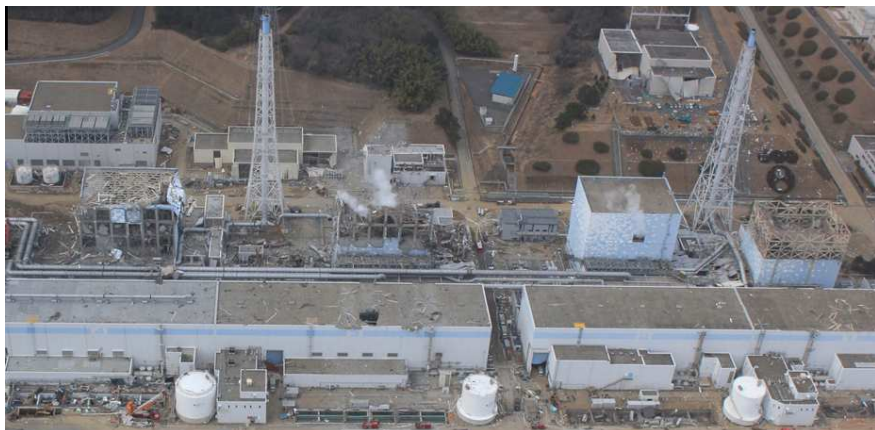
Figure 34. Picture of the Fukushima Nuclear Plant after the March 11 Japanese Earthquake and Tsunami Damage (Source: Grimston, 2011)
