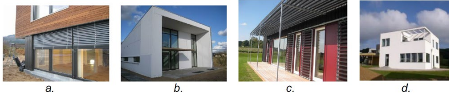
Figure 1. Four types of solar shading were analysed: a.) Integrated, b.) Construction as shading, c.) Manual shutters, d.) Patio.
