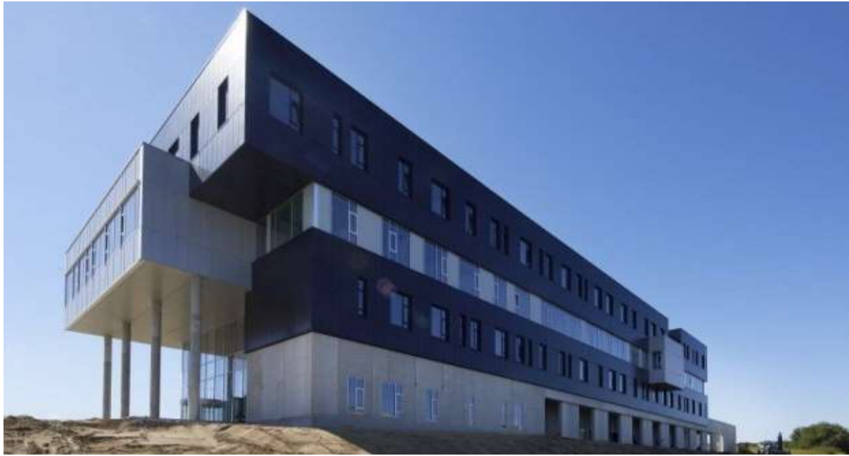
Figure 6: View of the North facade of the AAU-TMV building.
