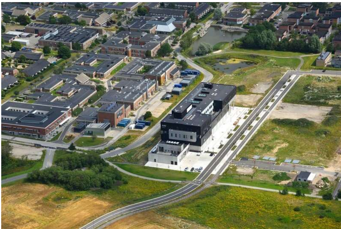
Figure 7: Aerial view of the AAU-TMV building in its surrounding environment on the Aalborg University main campus. The South façade, the West façade and the roof of the building are visible. In 2022, a new building was built on the East side of the AAU-TMV building (upper right corner of the AAU-TMV building in the picture) but was not visible yet in that aerial view. This new building on the East side of the AAU-TMV building was completed and opened on October 2022 ( https://www.aau.dk/grand-opening-e41542 ). The measurements on AAU-TMV were carried out in summer 2022, therefore, the external part of the building on the East side was already finished (credit to Aalborg University).
