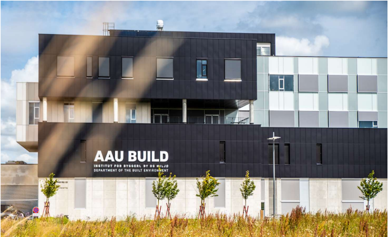
Figure 4: View of the South facade of the AAU-TMV building (credit to Aalborg University).
