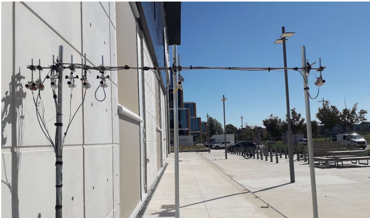
Figure 10: Air temperature measurement setup mounted on the South façade of the building.
