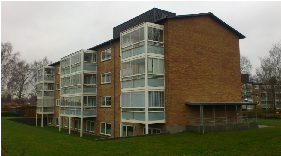
Figure 5.2. One of the renovated buildings. The ventilation units are placed on the roof. Also shown is the new glazed balconies.
