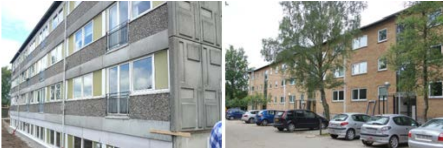
Figure 3. Photos of the building before (left) and after the retrofit.
