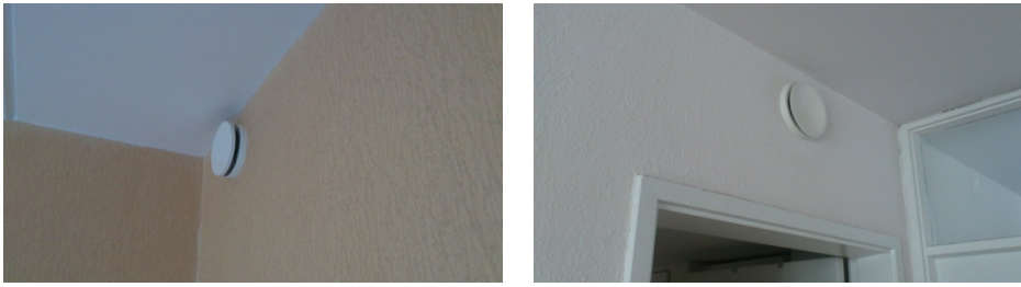
Figure 5.4. Examples of supply air terminals.
