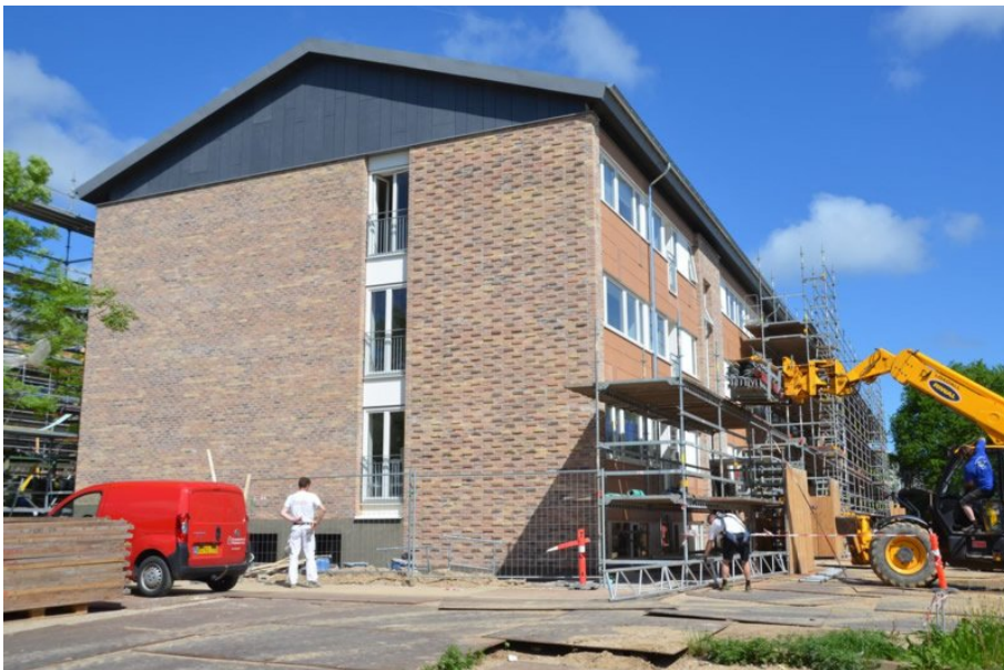
Figure 9. A new brick-wall end facade was erected outside the old end façade built on a new foundation. At the same time new French balconies were installed in the existing end facades. New tiles were attached to the old concrete construction on the entrance façade.
