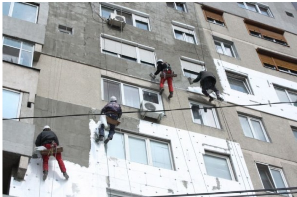
Retrofitting – blocks of flats
