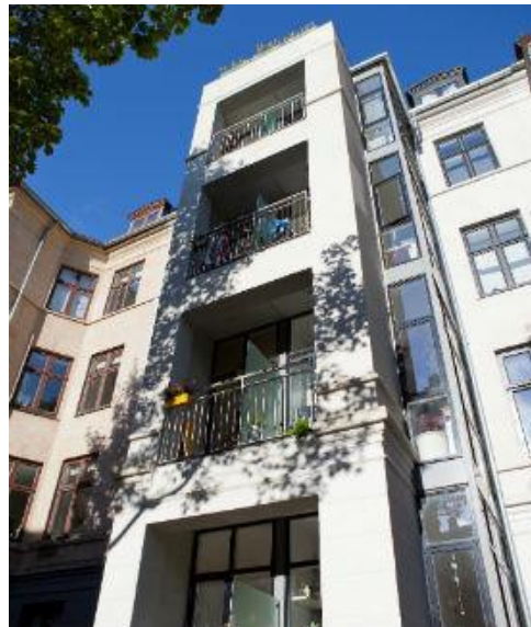
Copenhagen, exterior insulation and new balconies
