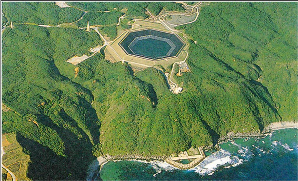
Figure 5-2: Photograph of a pumped hydroelectric storage facility using seawater [17].
