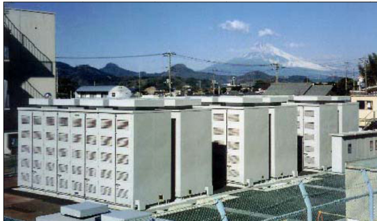
Figure 5-10: A 6 MW, 8 h sodium-sulphur energy storage facility in Tokyo, Japan [2].
