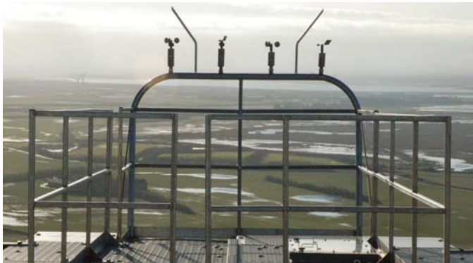
Figure 1 Arrangement of nacelle anemometry on the back of the nacelle of a modern wind turbines. The instruments are mounted on a reasonably solid support structure with lightning protection covering the instruments and with redundant mounting of cup anemometers and wind vanes
