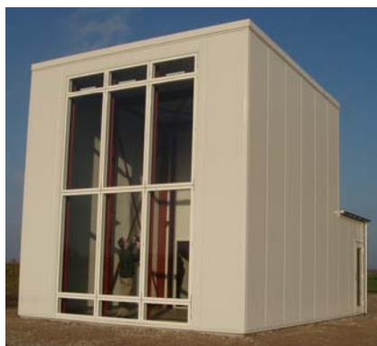
Figure 1. South (DSF) façade of the test facility.
