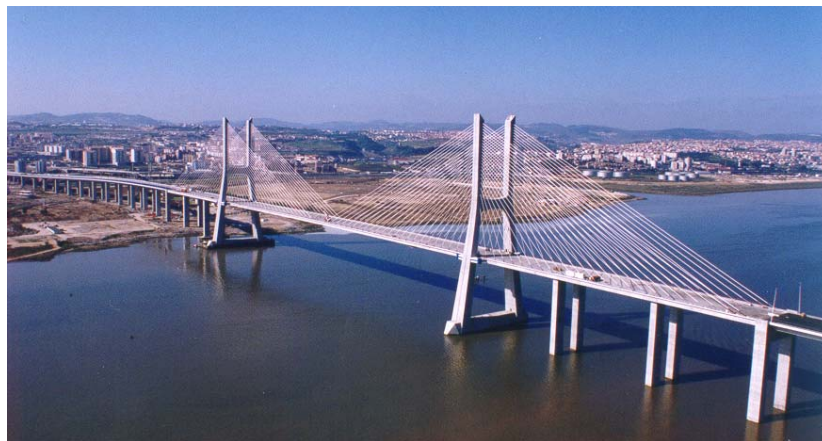
Fig. 1 – Cable-stayed component of Vasco da Gama Bridge
