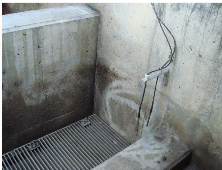
Figure 4. Water level switch for overflow indication
