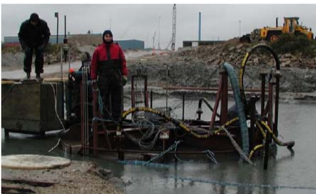
Figure 12. The 4x4m bucket successfully installed.
