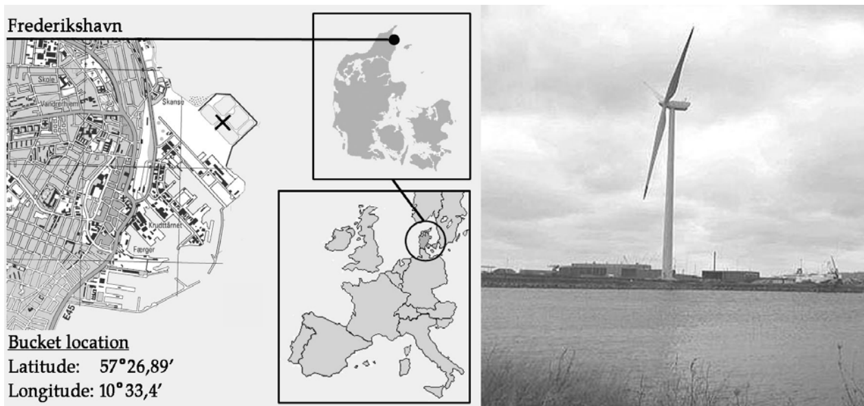
Figure 1. The suction bucket location and the Vestas V90- 3.0 MW wind turbine on the premises in Frederikshavn.
