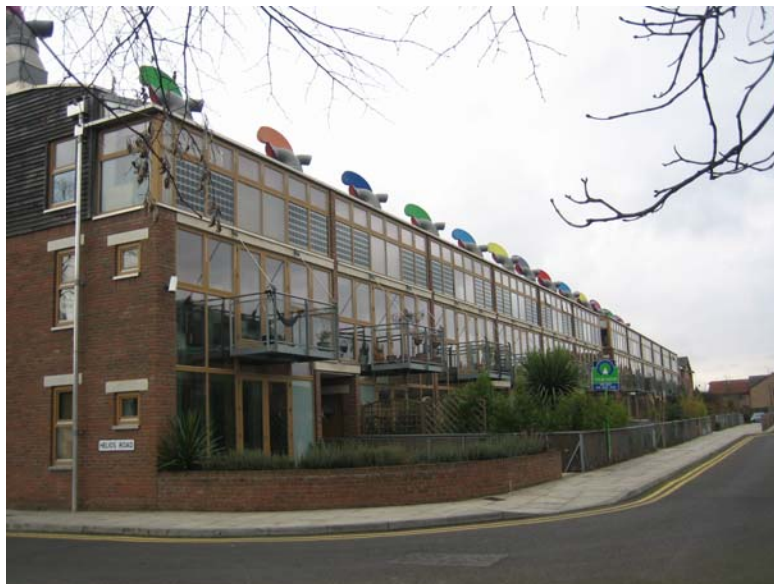
East facing façade with winter gardens and PV panels in the façade and on the glazed roofs of the winter gardens.
