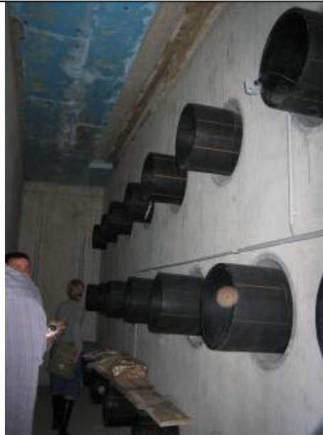
The picture shows the ducts through which the air is let into the basement area where the air is preheated or precooled.
