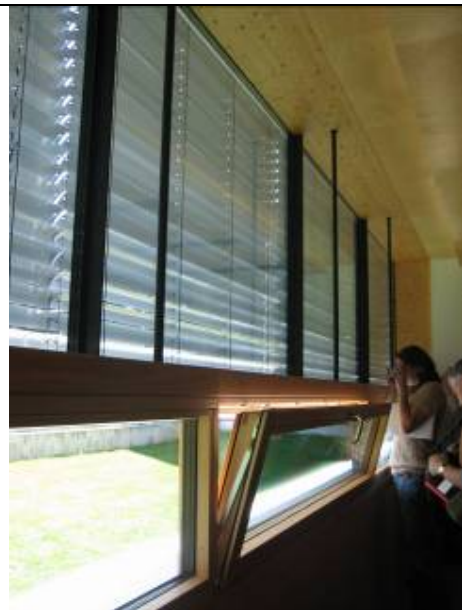
Picture of the façade in the classrooms. The external shading is automated, the automation can, however, be overruled by the users. Inlet openings are placed in the bottom in order to allow shading and ventilation simultaneously. The classrooms are also mechanically ventilated through inlet and outlet openings in the ceiling.
