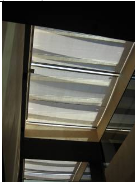
This picture shows the internal shading device in the atrium. The shading is activated when the temperature in the cavity is 40°C.
