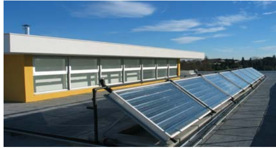
Roof window for ventilation and daylight and set of CPC solar collectors
