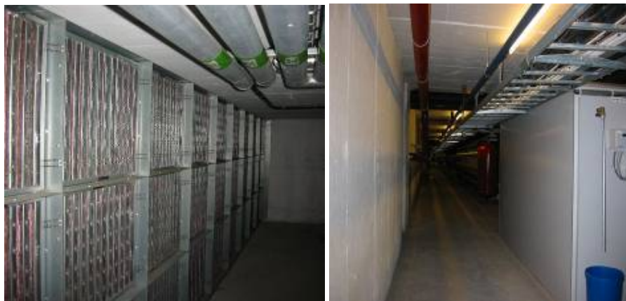
Filter at air intake in culvert (left) – low pressure drop. Storage tank for solar DHW is place in culvert (right). The culvert surfaces are painted.
