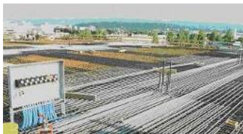
Installation of the TABS on site
