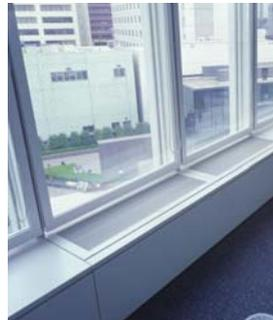
Figure 2.10b. Air Supply Swindow (View and detailed crossection)
