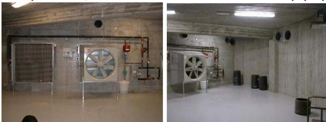
Figure 4.13. The air distribution room, showing the preheat unit (left) and fan, as well as the plastic subterranean ducts leading to the various rooms (Schild 2002a).
