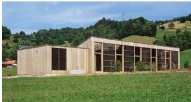
fig. 6.17: example of a house with PCM façade technology.
