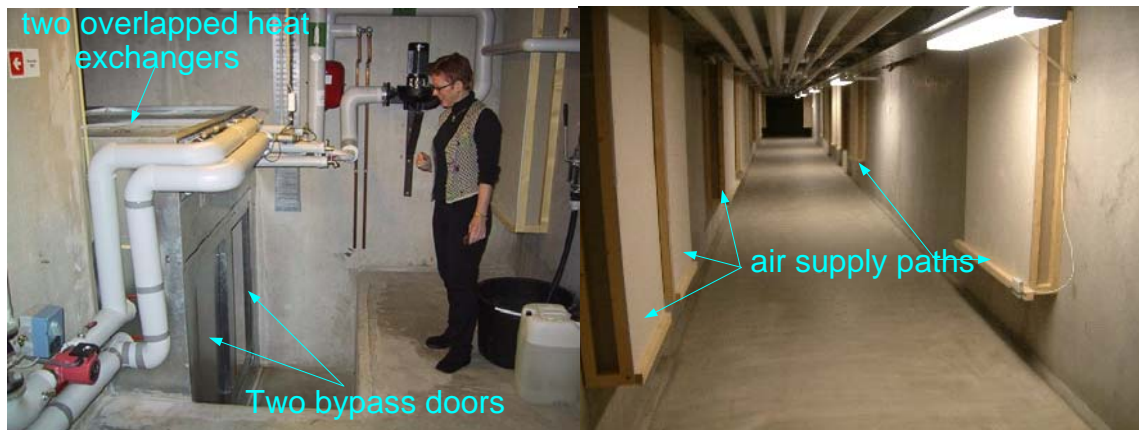
Figure 4.9. Air distribution duct of Mediå school (Left photo shows heat exchangers and “summer” doors. Right photo shows the supply air paths) (Tjelflaat 2002a).
