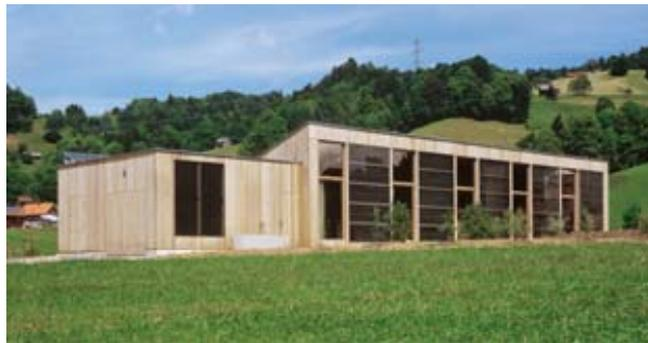
fig. 6.17: example of an house with PCM façade technology.
