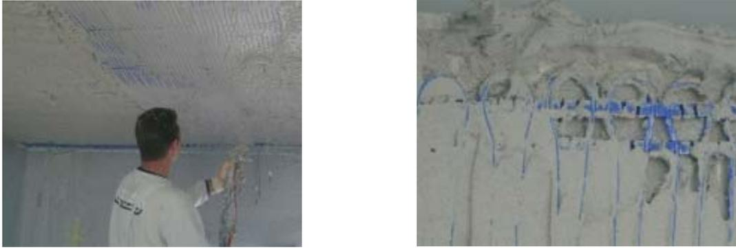
Fig.6.5: PCM plaster with integrated an hydraulic system (BASF).
