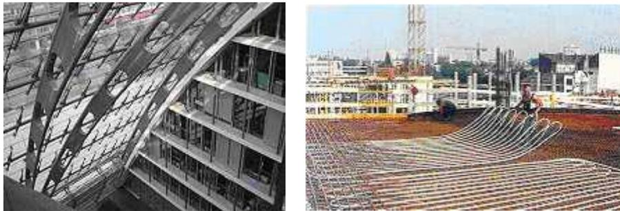
Figure 3.10 – Berliner Bogen: example of the building construction – double skin facade and floor slabs (left) where activating system of pipes was embedded (right) ([www.velta.de](http://www.velta.de))
