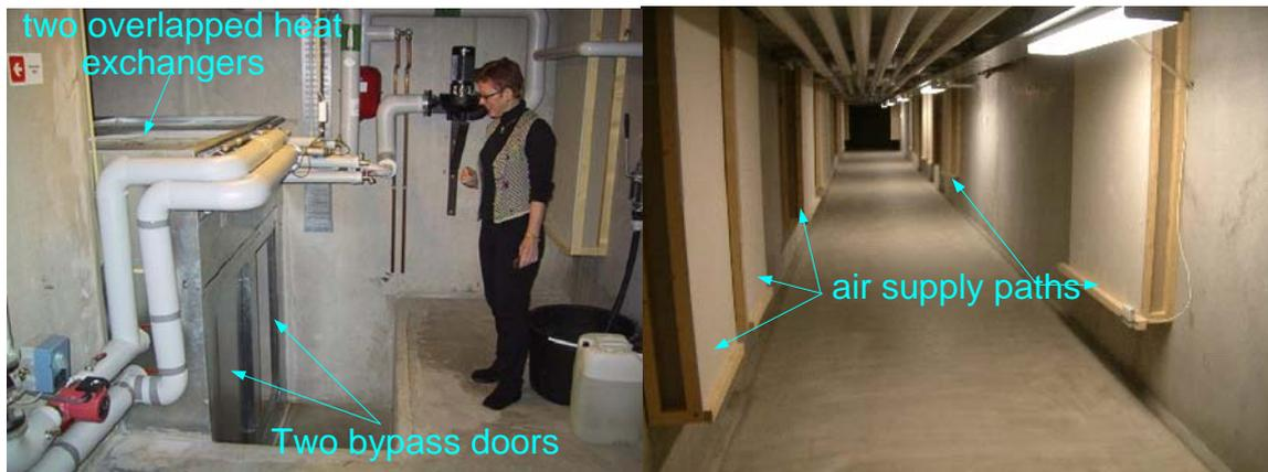
Figure 4.9. Air distribution duct of Mediå school (Left photo shows heat exchangers and “summer” doors. Right photo shows the supply air paths) (Tjelflaat 2002a).
