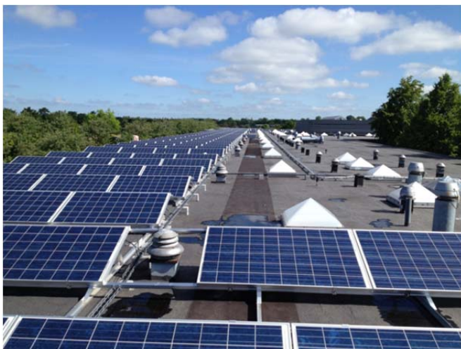
Figure 4. PV installation at Stengårdsskolen: 220 kWp – yearly production 173 MWh
