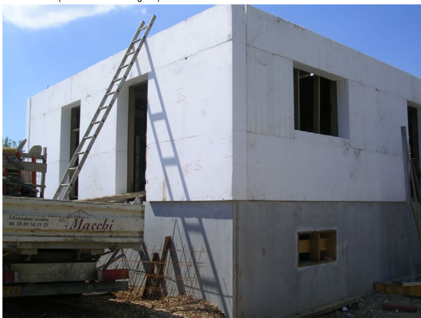
Figure 19: With prefabrication there is no more waiting period for interior paintings or the roughcast of the facades. (Foto: Frédéric Bougrain).
