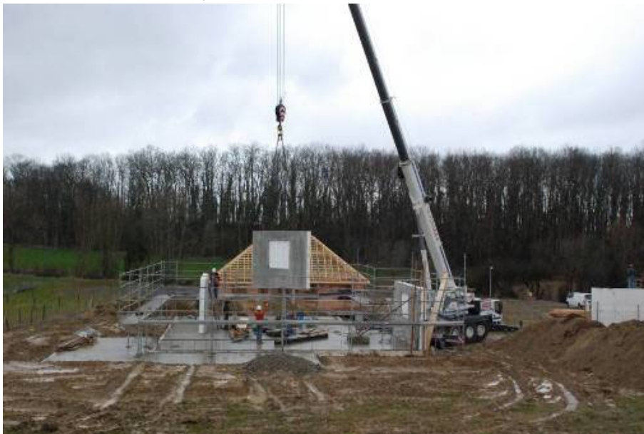
Figure 20: The use of cranes of strong tonnage to install prefabricated walls improves working conditions and reduces on-site risks. (Foto: Frédéric Bougrain).
