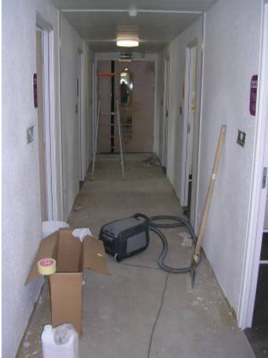
Figures 27: Renovation works. (Foto: Frédéric Bougrain).
