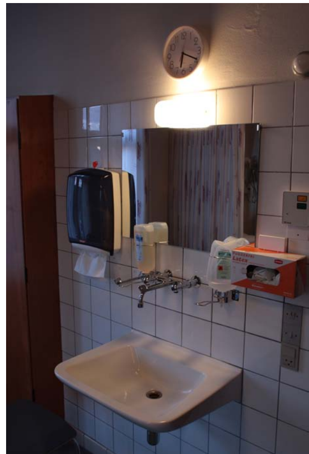
Figure 18: Hospital sink in artificial light.
