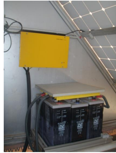
Fig. 5. Detail of the interior view of an FSA, including a set of batteries and its charger.
