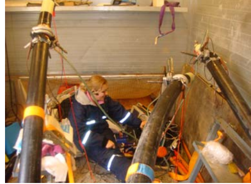
Fig. 9 Measurements performed on an open end of the 150 kV land cable
