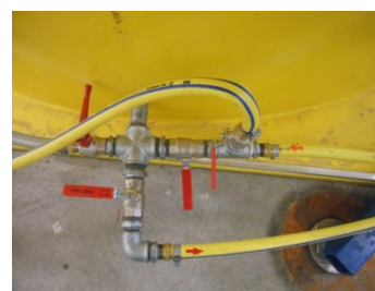
Figure 2. In and out flow valves.
