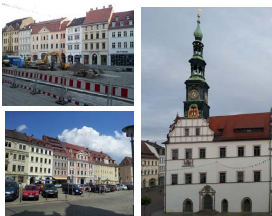
Figure 1. Façade restoration work in the German cities of Zittau (upper left), Görlitz (lower left), and Pirna (right)
