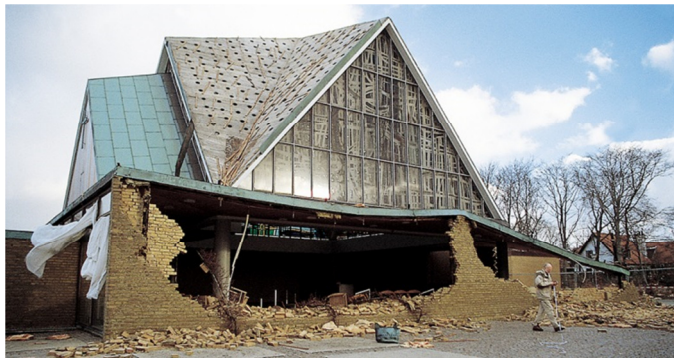
Figure 2. Damage to a building after the heavy windstorm passed over the southern half of Denmark on 3 December 1999.
