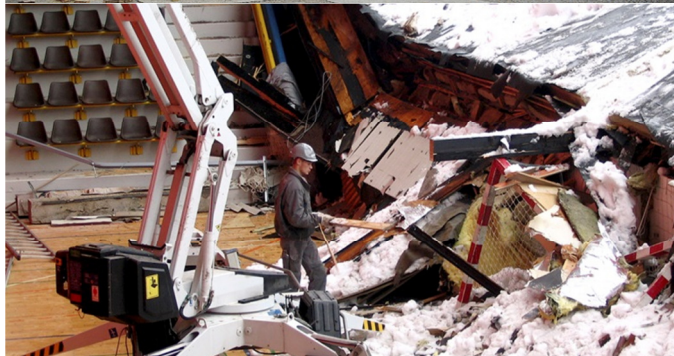
Figure 3. Damage to a sports arena after the roof collapsed, caused by heavy snow loads in 2007.
