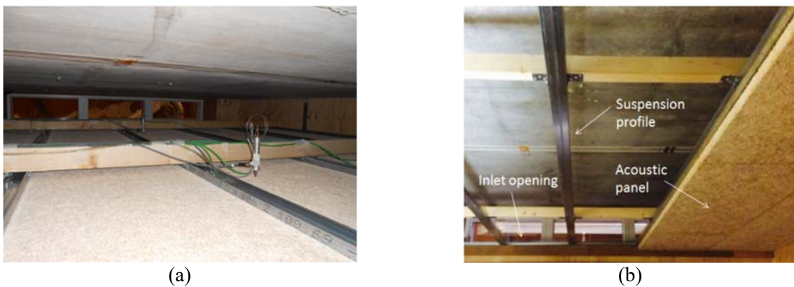
Figure 10: Overhead plenum and diffuse ceiling setup [4]
