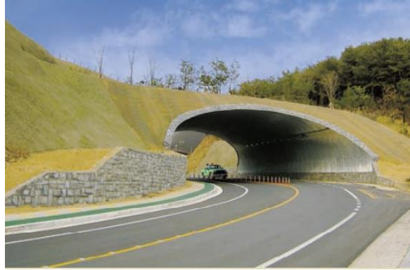
Figure 2. A steel soil composite bridge [19]
