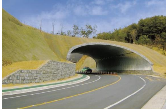
Figure 2. A steel soil composite bridge [19]
