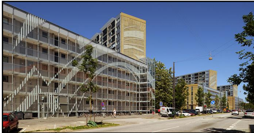
Figure 2 Focus on transparency for the renovation of a residential building in Copenhagen, by Pålsson Arkitekter A/S, and making the inhabitants feel safer (by using stair towers covered with glass) and proud, where the street picture is improved. The glass facade is historically inspired from an old stream that was in the area.
