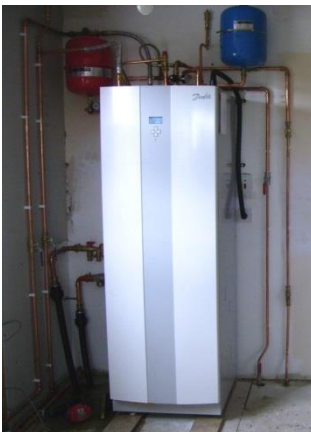
Figure 42. Heat pump with its connection pipes.
