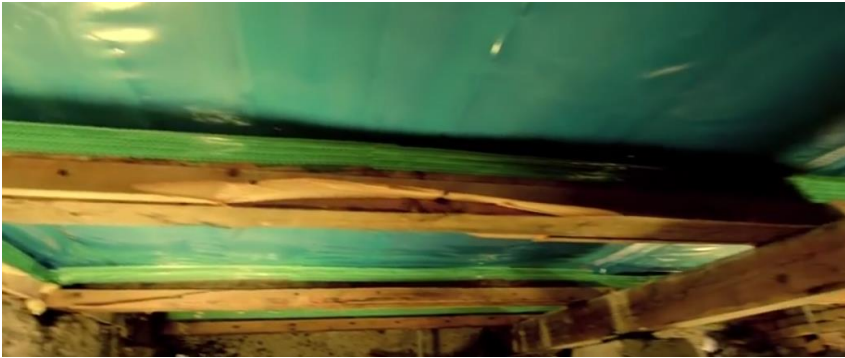
Figure 55. Vapor membrane under existing wooden floor above crawl basement.
