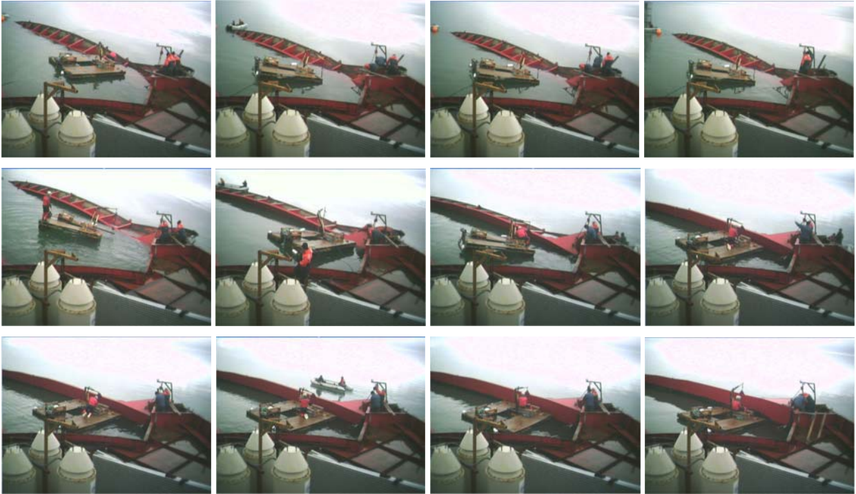
Figure 7.2. Reinstallation of starboard reflector after dislocation, occurring between Christmas and New Year 2003.
