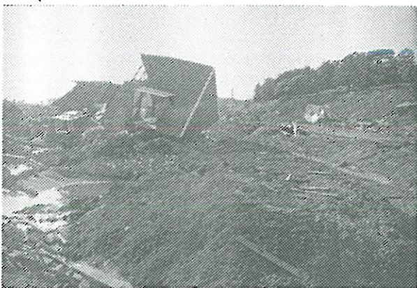
Fig. 29 The dire result of the presence of quick clay, Tuve Sweden.
