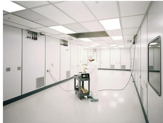
Clean room with piston flow (Shelco Inc).
