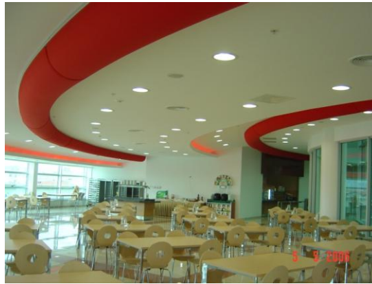
Figure 4. Vertical ventilation from openings in the ceiling. a_o/A \sim \text{medium} . The photo shows this type of flow from ceiling mounted textile terminals (KE Fibertec A/S).
