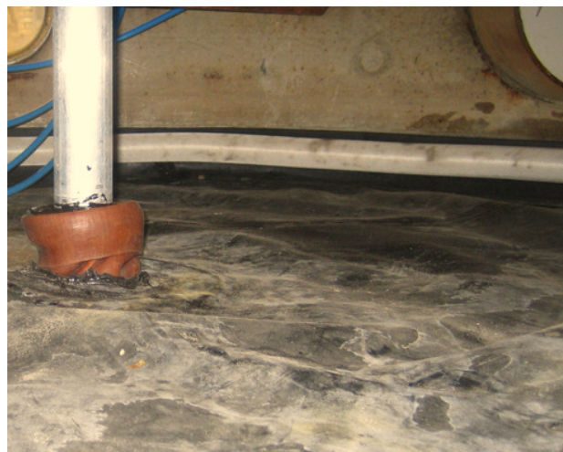
FIGURE 4. MEMBRANE PLACED ON TOP OF THE SOIL.
