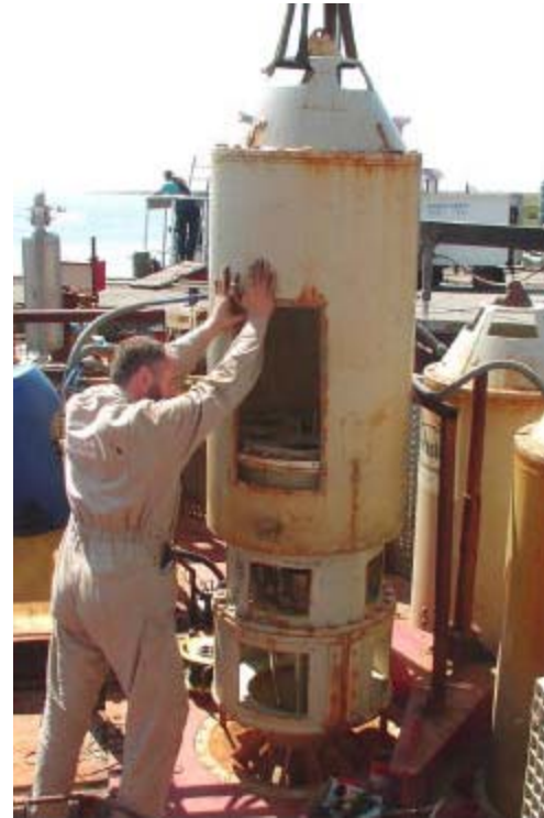
Figure 11: Reinstallation of turbine.
