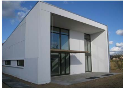
Figure 3.15: Solar shading in house 45.
