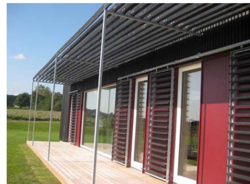
Figure 3.11: Solar shading in house 39.
