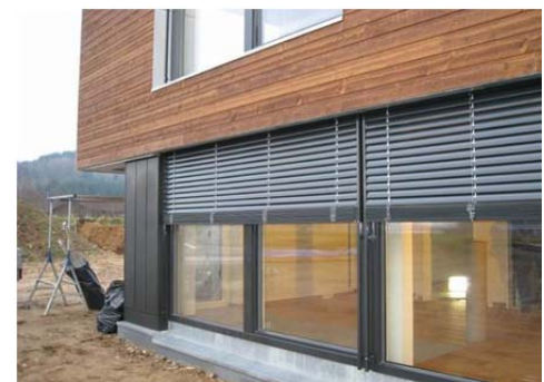
Figure 3.13: Solar shading in house 43.
